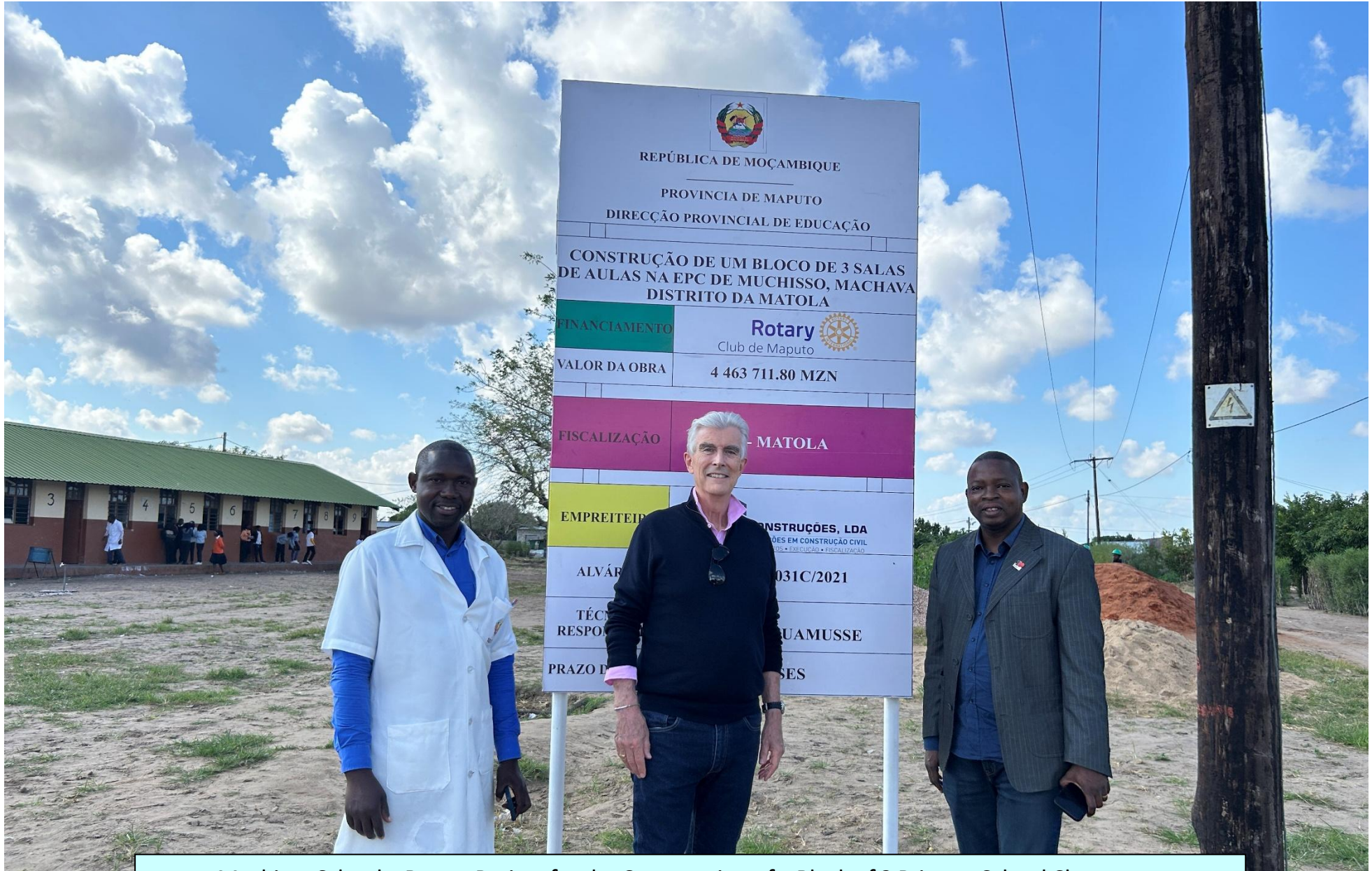
Machisso School – Rotary Project for the Construction of a Block of 3 Primary School Classrooms
